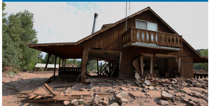
Flash flooding following the Hayden Pass Fire caused extensive property damage in the Coaldale community. Actions proposed by Colorado Headwaters would help mitigate the destructive effects of wildfires.
